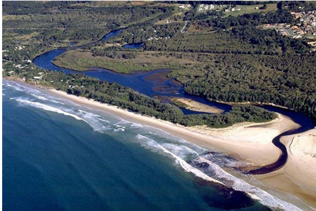
Belongil Creek outlet operating after a rain event.
